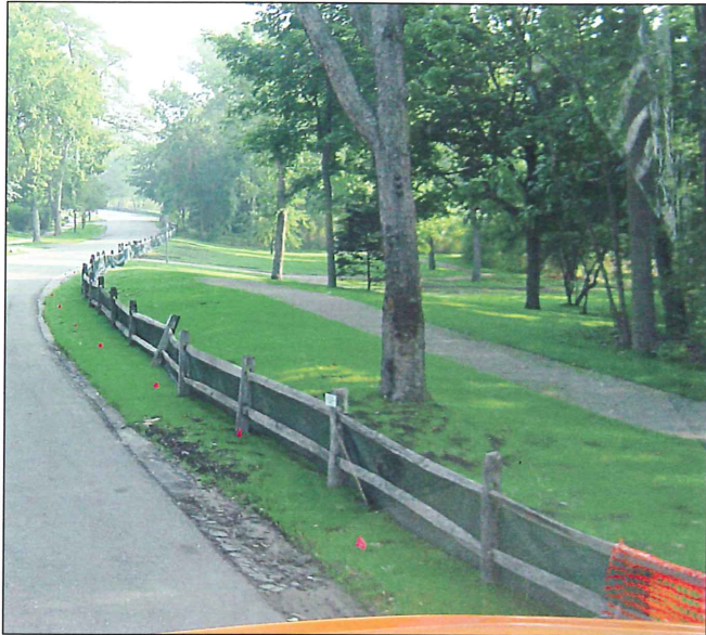
The turf restoration process (pneumatic conveyance) that Doetsch Industrial Services, Inc. used on the Quarton Lake project in Birmingham yielded significant vegetation growth in only a matter of about 15 days after applied.
