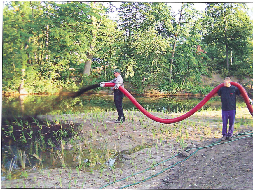
TOP: Mike Mehal (left) and Don Landis (right) apply the compost to a vegetated wetland by pneumatic conveyance at Quarton Lake. The process did not disrupt the existing plants at any point. RIGHT: Doetsch had completed the actual conveyance of the compost at Quarton Lake by the end of July 2003. BOTTOM: Dave Black (left) and Jason Hale (right) gradually uncover and expose a massive underground configuration of pipes and wires by using hydro-excitation.
