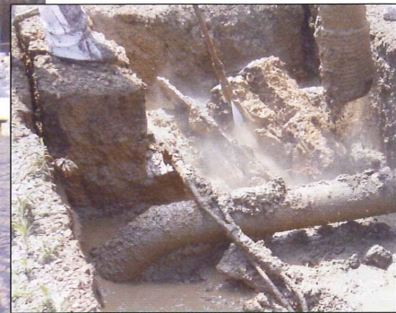
At the left, hydroexcavation created a 1,200-foot-long trench for an electrical conduit run for a Michigan utility company. Above, location of direct burial electrical wire using a 15 degree fan tip nozzle at 10 gpm.
