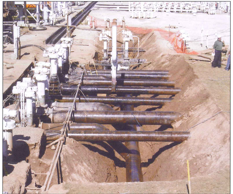
Hydroexcavators perform a mass excavation of a pipe repair pit.
