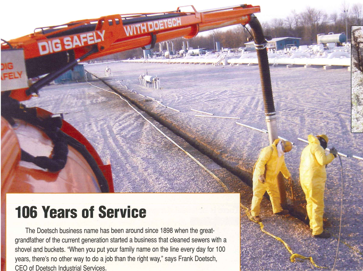
At the left, hydroexcavation created a 1,200-foot-long trench for an electrical conduit run for a Michigan utility company. Above, location of direct burial electrical wire using a 15 degree fan tip nozzle at 10 gpm.
