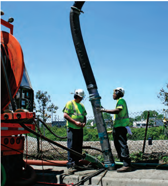
Crew uses vector to clear the Sharkey Drain siphons.
