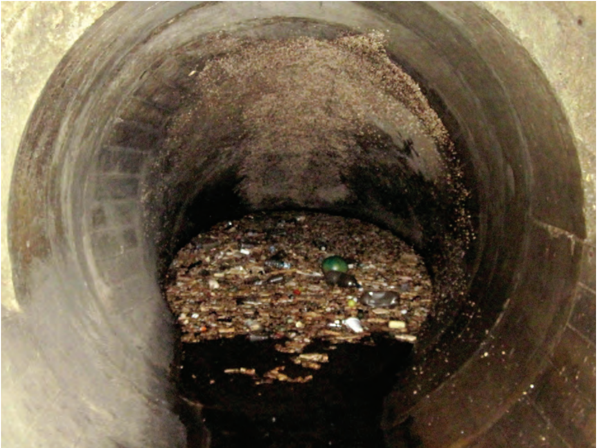
Pre-project conditions in Sharkey Drain, under I-696 in Macomb County.
