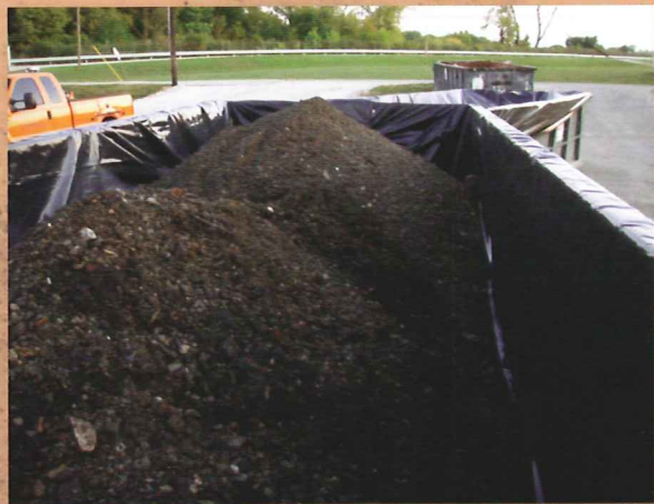
Debris packaged for the landfill
